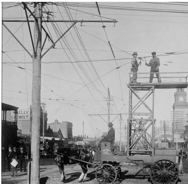
Tower erection at Kalgoorlie Electric Tramways, 1902.
