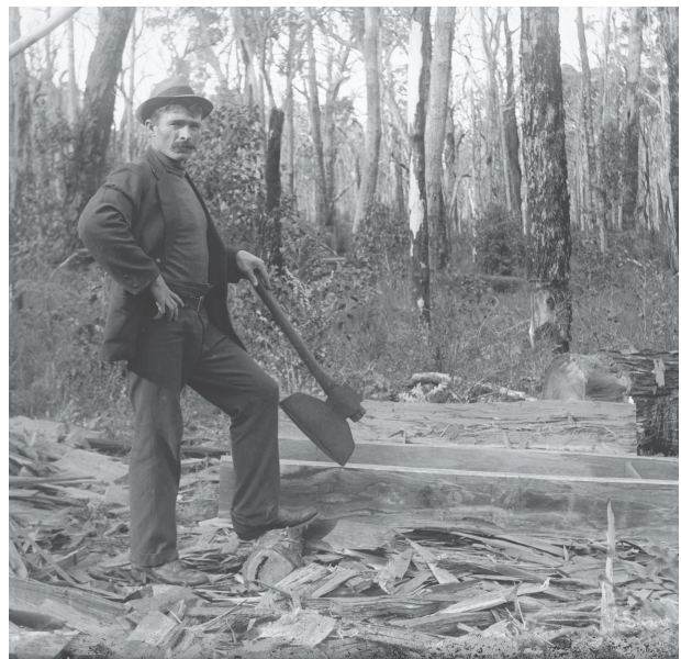
Sleeper cutter with broadaxe, c1920s.
