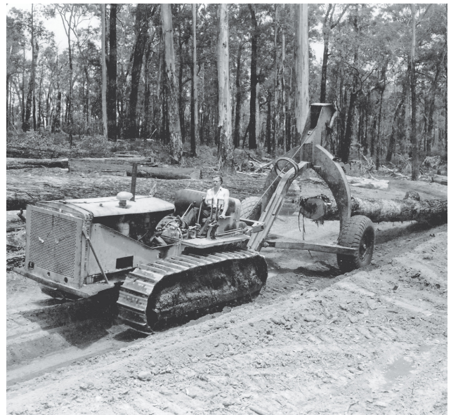
Rubber Tyred Arch Courtesy State Library of WA 816B/TBt337
